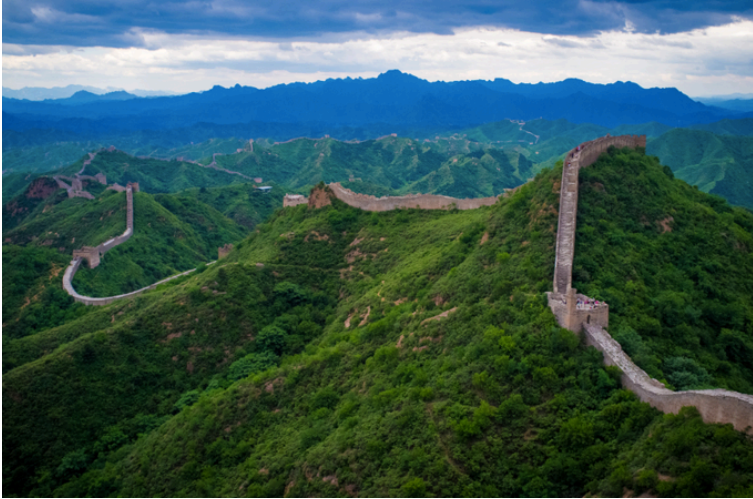
The Great Wall of China.
