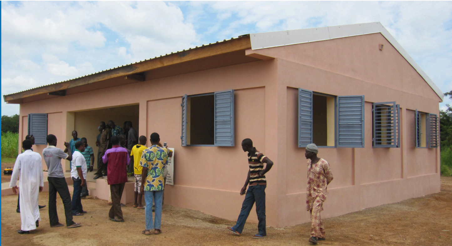
Figure 17.1 The US Army Corp of Engineers opened this community health clinic in the country of Benin in West Africa in 2013. The clinic has waiting, consultation, observation and treatment rooms, and a drug store. (credit: “Pehunco Health Clinic opens” by US Army Corps of Engineers/Wale Adhlakun/flickr, Public Domain)
